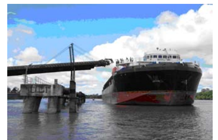
12,000 dwt self-propelled barge berthing at Kelanis
