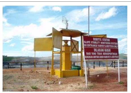
Slope monitoring by robotic theodolites
