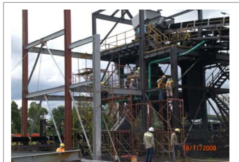
Installation of the new crusher system underway at Kelanis
