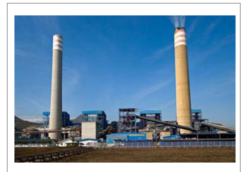
PT Paiton Energy's 1200 MW plant was the largest consumer of envirocoal in 2008
